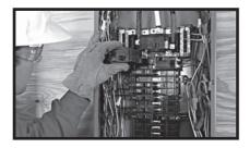
Install a 2-pole breaker in the distribution panel to protect the transfer switch. The required Amp rating of the breaker depends on which transfer switch you're using, so refer to the Installation Guide before purchasing the breaker.
